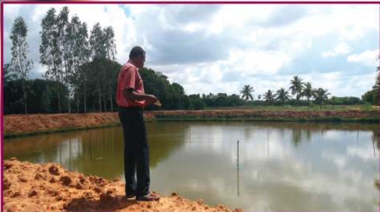
Dist Govt . officer from DWDA. Pudukkottai inspecting the works ( After rain)
