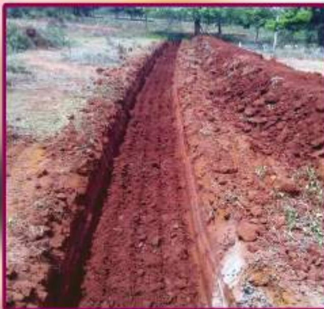
Executed Field Bunds ( Before rain )
